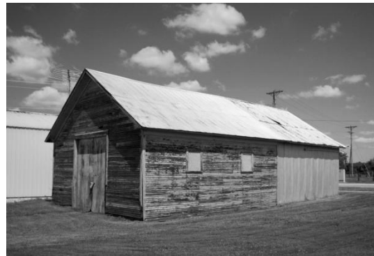
Bulk Oil Station Building along railroad grade at 505 Scott Street
