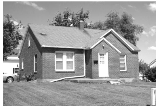
816 South First Street
