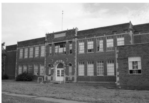
Washington School 509 East Harrison Street
