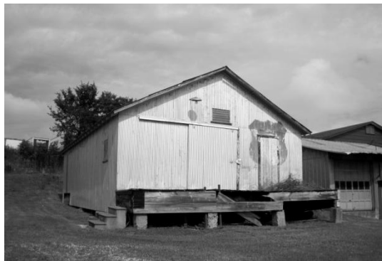
Bulk Oil Station Building along railroad grade at 903 Green Street
