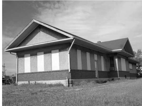
Quincy, Omaha and Kansas City Railroad Depot, 904 North Elson Street
